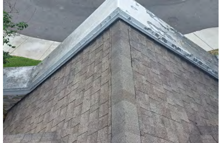
Front Porch Gable Wall Capping
